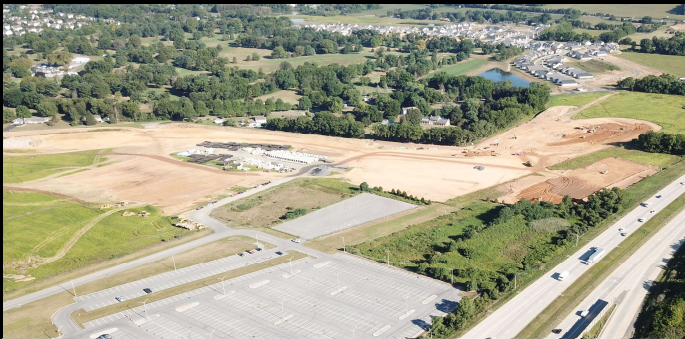
Easton, PA | 500,000 SF Flex | Under Construction
